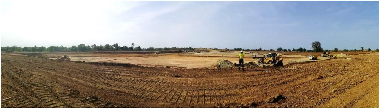
Figure 4: Surface Water Management Pond under construction
