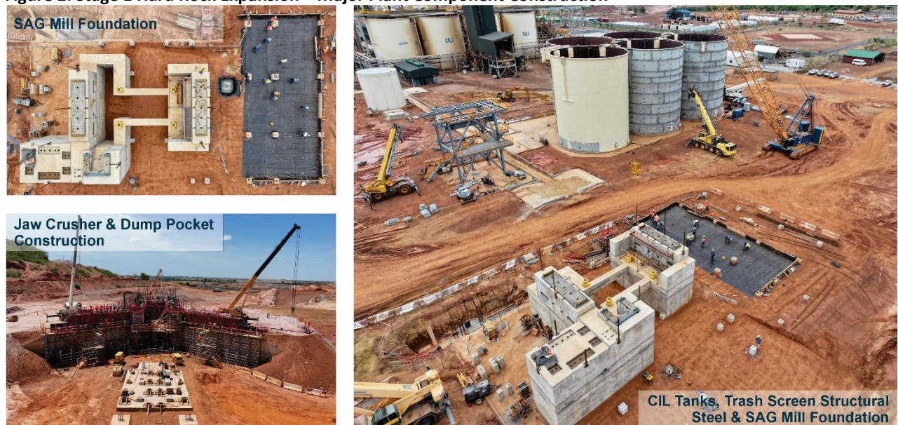
Figure 2: Stage 1 Hard Rock Expansion – Major Plant Component Construction
